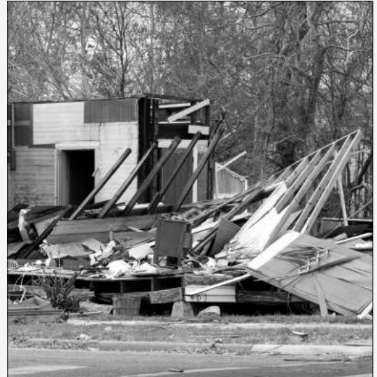
Hurricane Ivan's powerful winds destroyed homes in Pensacola, 2004.
