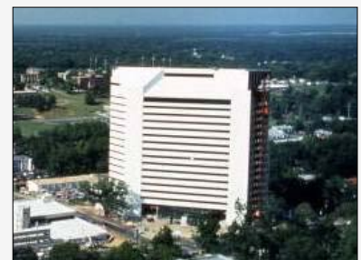
Turlington Building Florida State Archives
